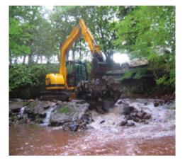
more distant point upstream. The construction of the weir was typical of that era: dressed stone fitted into a robust wooden framework and blockstone crest. The fact that the frame was still there along with a series of 'generational' concrete repairs might have suggested a larger machine would be needed but the 10 tonner used eventually completed the task.
