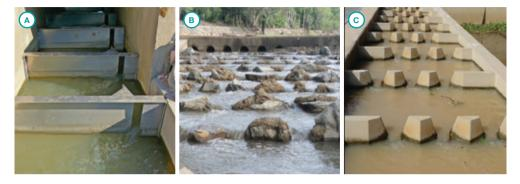
(25-30 W/m<sup>-3</sup> [Cd 0.7]) vertical-slot fishways and fish locks are used; either with small pools dedicated for small fish or larger designs to also pass large fish. At sites with small headwater fluctuation, rock-ramp fishways and cone-baffle fishways are widely used, as well as roughened sides of culverts (Amstaetter *et al.*, 2017).
